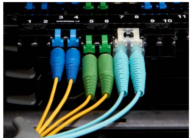
Adapter packs accept a variety of connector types
