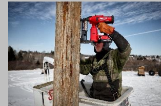
Using bucket trucks to mount wire to vertical pole
