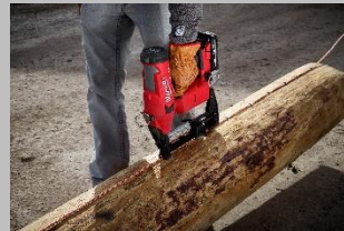
Installing wire before pole is upright
