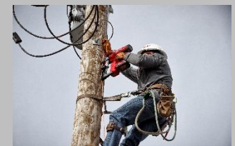
Climbing pole to install wire
